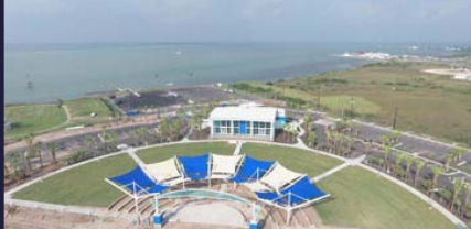
Cameron County Amphitheater & Events Center - Photo by Cameron County Parks & Recreation
