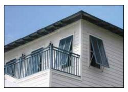
Figure 4-10. Bahama shutters made from durable extruded aluminum components add "Island" flair to a home and provide opening protection.
