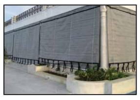
Figure 4-16. Polyethylene basket-weave fabric windscreen is deployed at the edge of a patio, enclosing the entire area.
