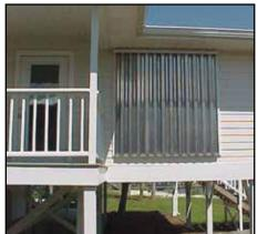
Figure 4-13. These 0.050 gauge aluminum storm panels offer cost-effective storm protection. In this example, panels slip into a track above the window and secure onto a bottom track using wing nuts.
