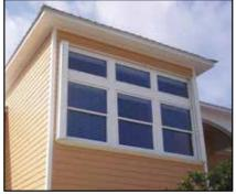
Figure 4-9. Accordion shutter (shown in open position) installed over a large window group of a coastal home. Shutter has been installed to allow deployment from inside the home.
