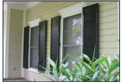
Figure 4-11. Colonial shutters made from durable extruded aluminum components add a traditional look to the home and protect window openings.
