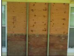
Figure 4-19. For larger windows, such as this sliding glass door, two 2x4s face outside and are oriented with the narrow end against the plywood. The fastening screws attach from the plywood into the 2x4.
