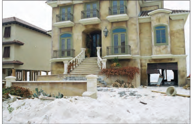
Large solid stairs such as these block flow under a building and are a violation of NFIP free-of-obstruction requirements.
