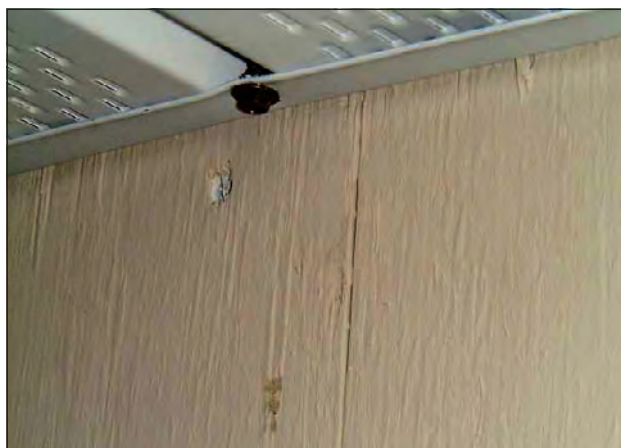
Figure 5. Screws through wall channel.
