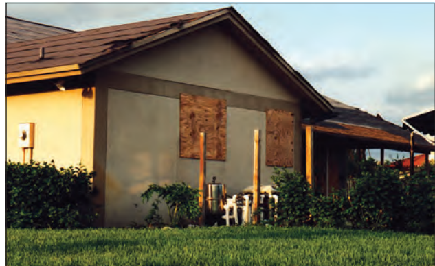
Figure 1. Wood structural panels installed in accordance with building code requirements are a cost-effective means of protection, but they should be adequately attached so they themselves do not become windborne debris.
