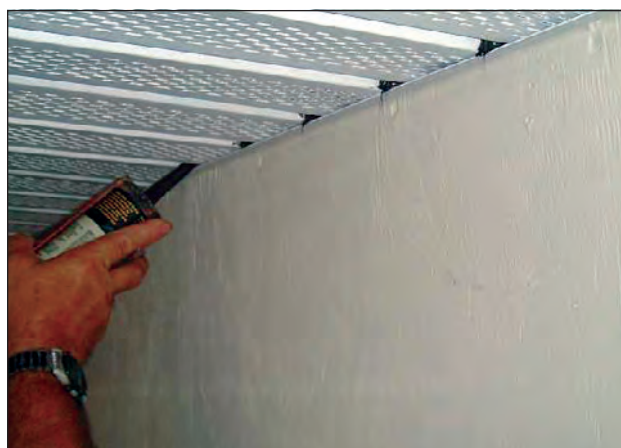
Figure 4. Applying dabs of sealant.
