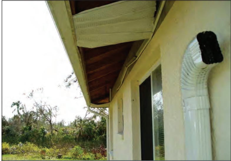
Figure 1. Missing soffit material.
