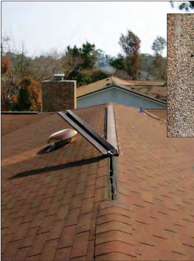
Figure 8. This metal ridge vent was attached with widely spaced roofing nails.
