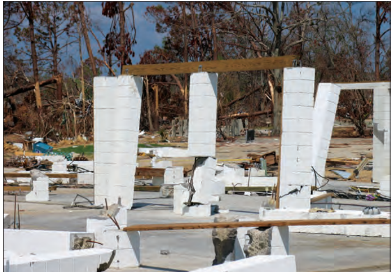
Figure 2. Pier breakage (Long Beach, Mississippi)
