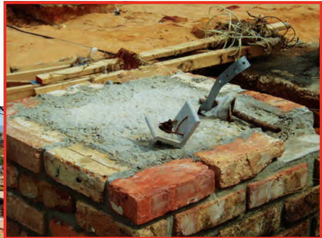
Figure 3. Failure of pier-to-beam connections due to wave and flood forces acting on the elevated building (Long Beach, Mississippi)
