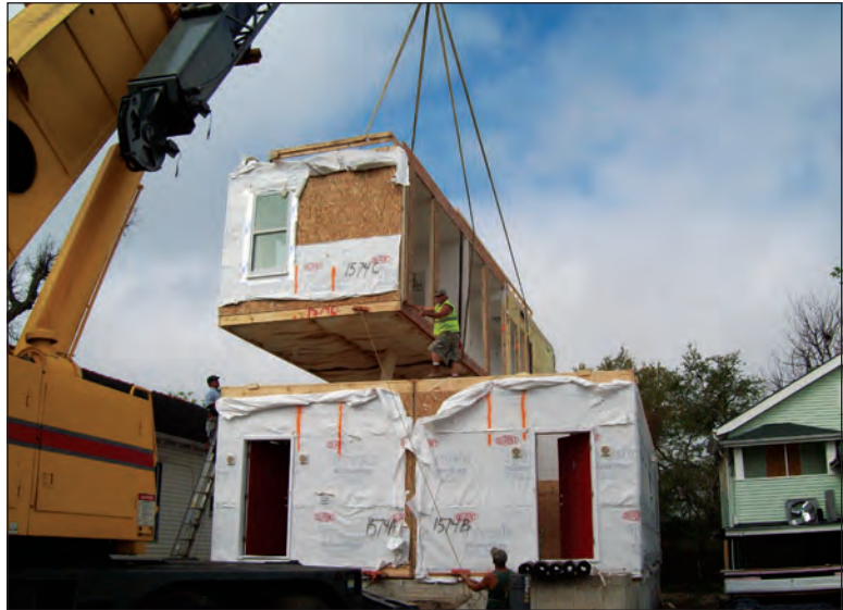
Figure 1. Construction of a modular home.
