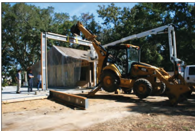
Figure 4. Installation of a prefabricated ordinary moment frame.
