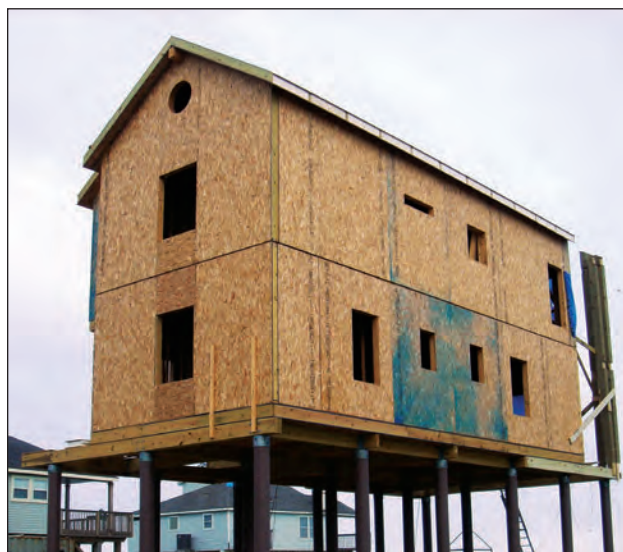
Figure 2. Construction of a Structural Insulated Panel house.
